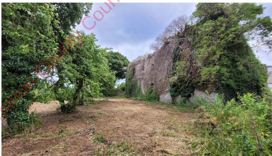
Image 4-3: Old stone structure and old orchard to the east of the site
